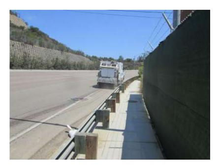
**Photo 4:** A street sweeper cleans paved roadway surfaces adjacent to the project site to remove trac-out in accordance with the SWPPP and MM-HYD-1.
