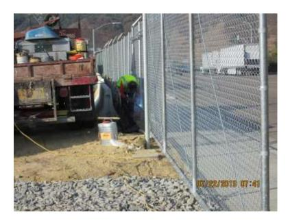
**Photo 5:** Fire suppression equipment consisting of a fire extinguisher and backpack pump was on site during welding activities in accordance with Mitigation Measure HAZ-2.
