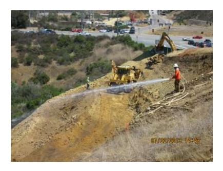
**Photo 3:** Water is utilized in areas of active construction to minimize fugitive dust emissions.
